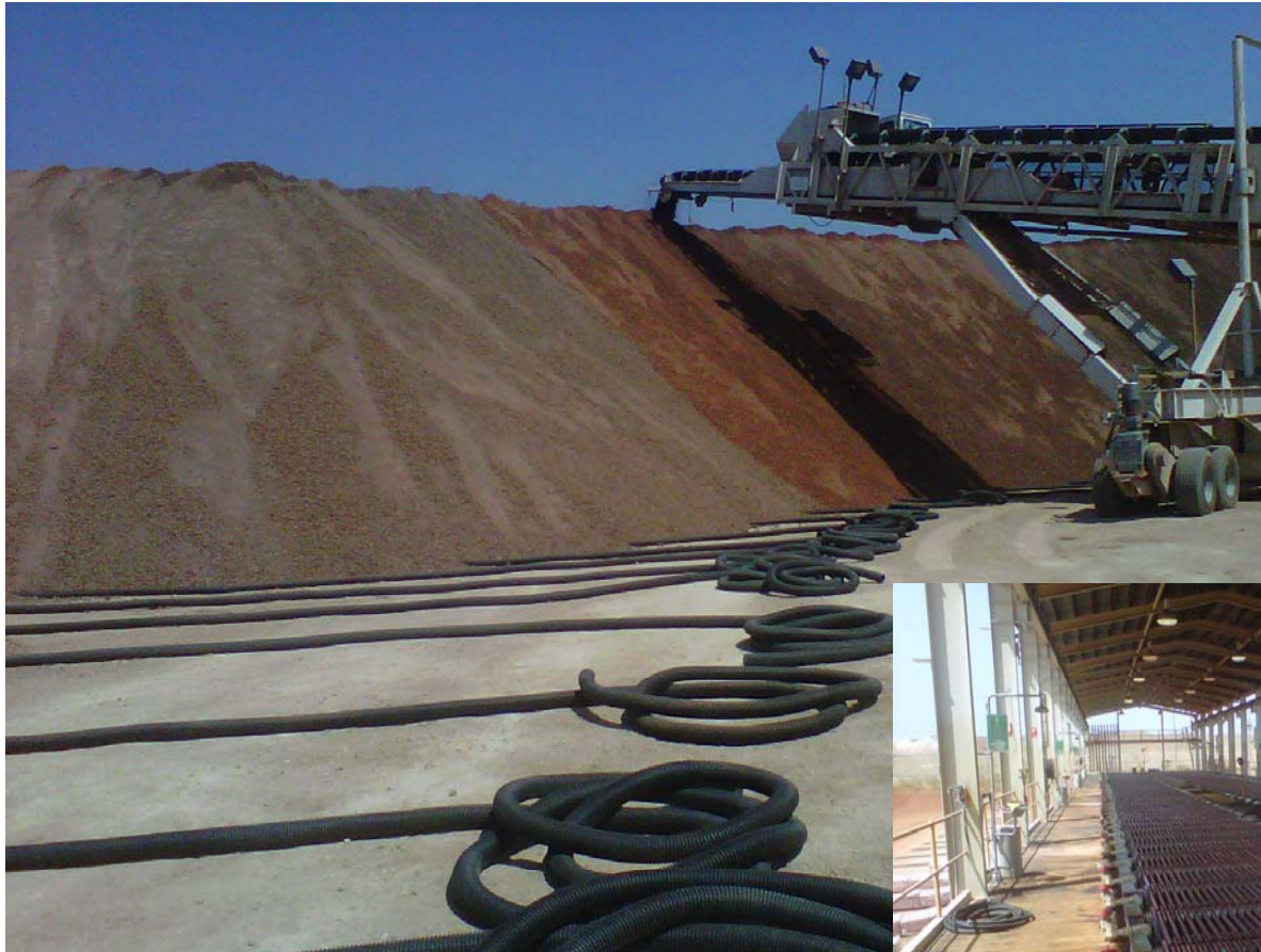
Pad Construction Design 4-6m lifts
